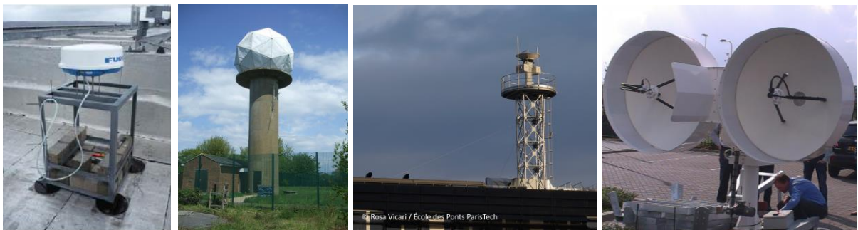
Figure 2. Radars implemented at the pilots sites of RainGain (from left to right): X-band single pol radar implemented in Leuven, Chenies C-band radar of the UK national network, dual-pol X-band radar installed in Paris, dual-pol X-band radar to be installed in Rotterdam.
